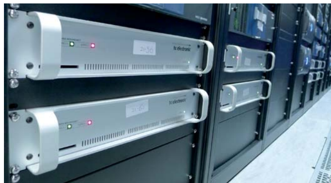
20 TC Electronic DB8 MkII processors are dedicated to transmitting the audio in each of the five control rooms
